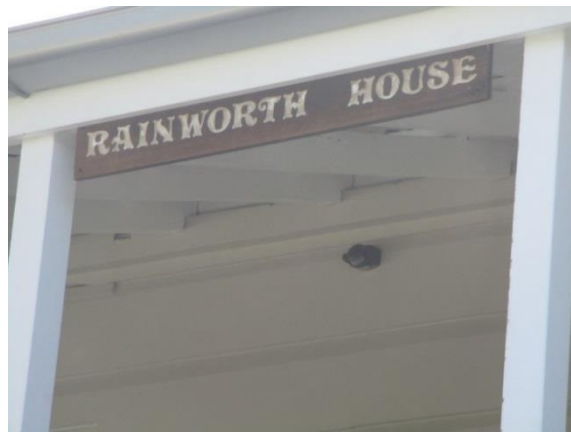
The re-instated name of " Rainworth House ".
