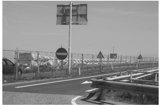
Stockpiled protection concrete blocks behind a barrier fence at The Afsluitdijk stopping point. This material will be used to raise the dyke level.
