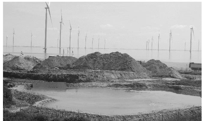
Current earthworks associated with raising the Afsluitdijk Dyke.
