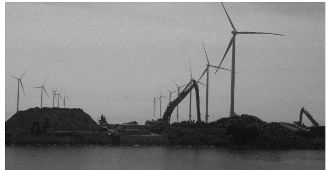
Current earthworks associated with raising the Afsluitdijk Dyke.
